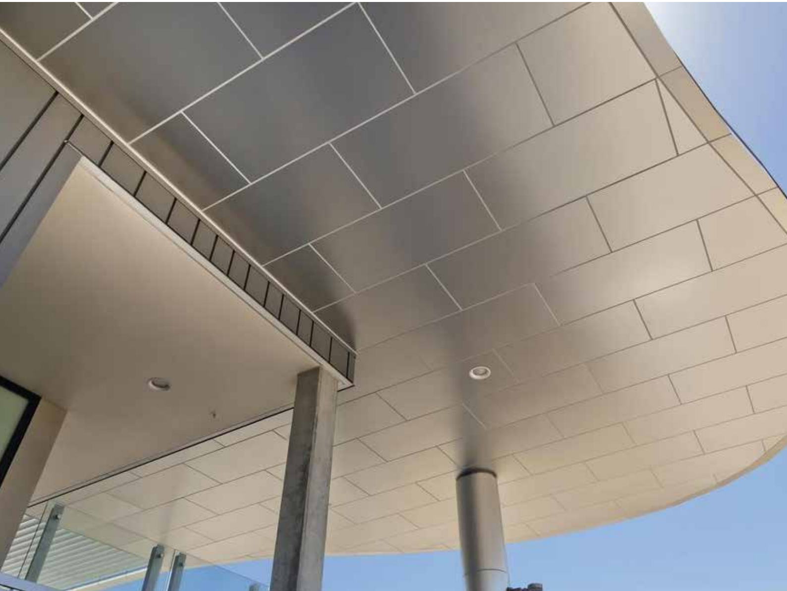
SDCCD Mesa College Social and Behavioral Science Building, San Diego, California (USA) - Architect: Joseph Wong Design Associates - Technique: VMZINC® Interlocking profile.
